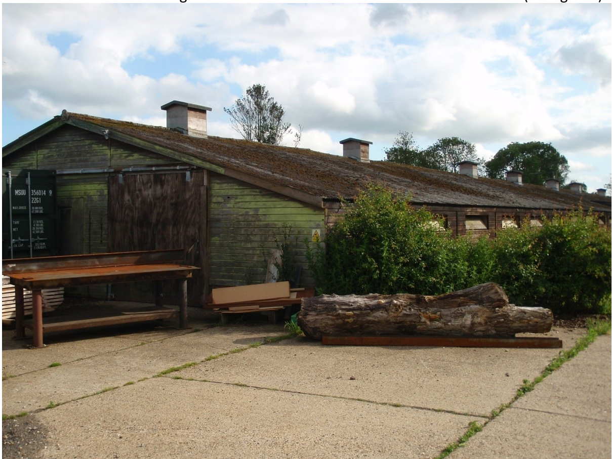
Plate 10: View of the north western corner of the eastern most barn (facing SSW)
