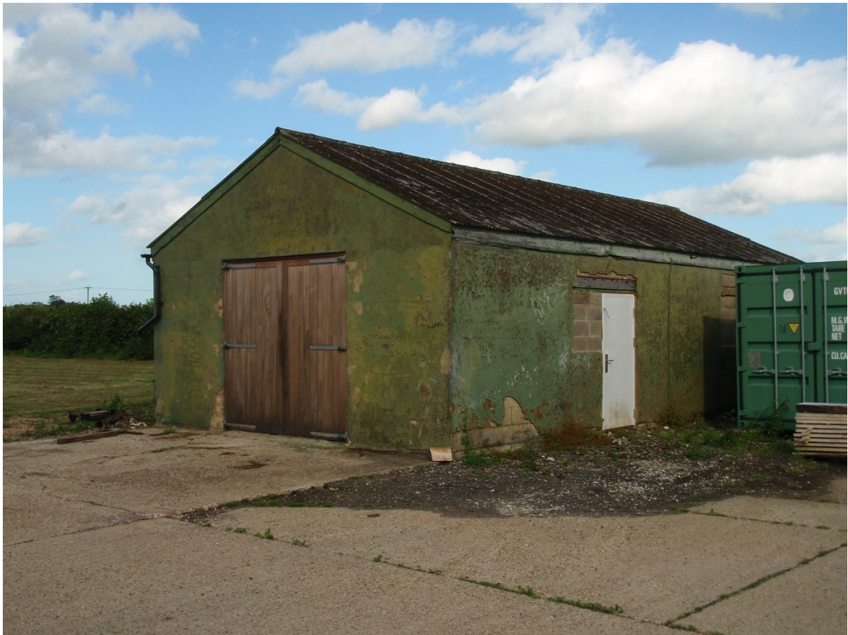
Plate 9: View of the building at the north eastern end of the eastern most barn (facing ENE)
