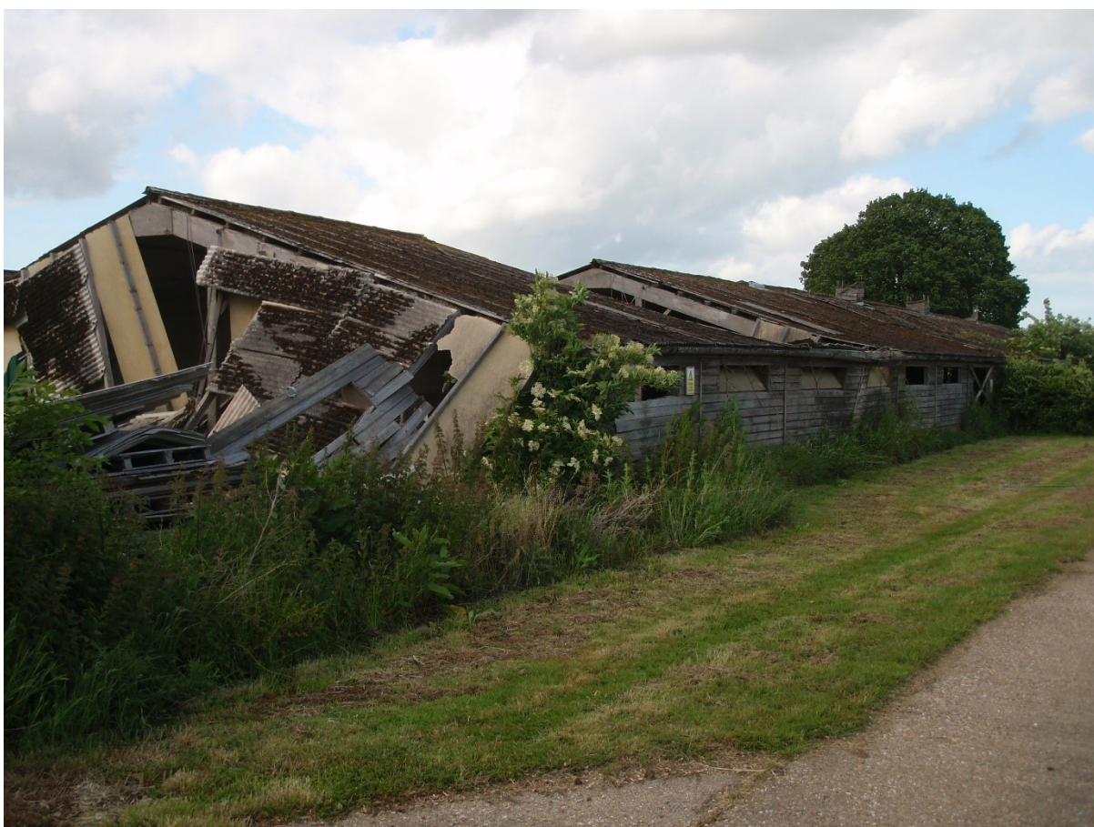
Plate 8: View of the western barn building (facing NNE)
