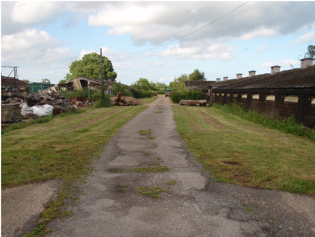
Plate 7: View across PDA (facing NE)
